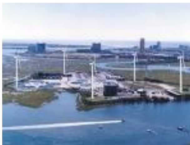
The Atlantic City wind farm. Five AFT rated at 1.5 megawatts each. The height with a blade in vertical position is 380 feet.
